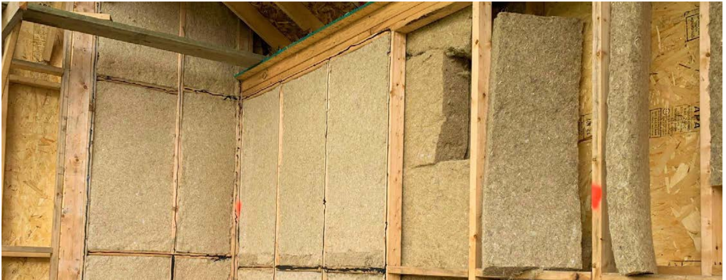
Photo 1. Installed Natur-Chanv/Hemp™ insulation panel
